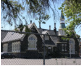
PRIMARY SCHOOL NO.253 SOHE 2008
