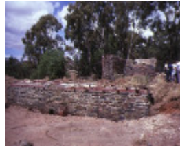
1 north british gold mine parkins reef road maldon side view dec1984
