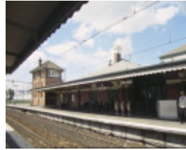
footscray railway station complex irving street footscray centre platform view sep1998
