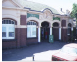
footscray railway station complex irving street footscray front view dec1985
