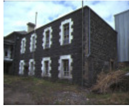
henderson house footscray bluestone building
