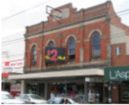
FORMER BATES BUILDING SOHE 2008
