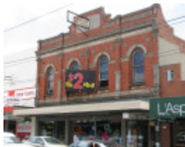
FORMER BATES BUILDING SOHE 2008
