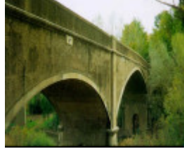
bridge over moorabool river fyansford front elevation publication
