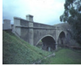
1 bridge over moorabool river fyansford side view jul1984
