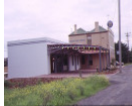
fyansford hotel fyansford rear view
