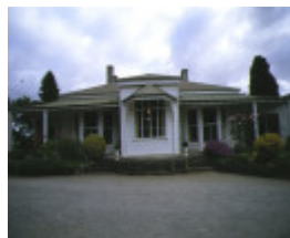
1 the heights 140 aphrasia street geelong front view homestead apr1997
