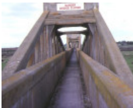
barwon river ovoid sewer aqueduct barwon river geelong view of top aug1988
