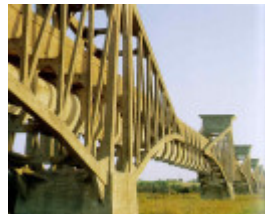
barwon river ovoid sewer aqueduct barwon river geelong site view publication
