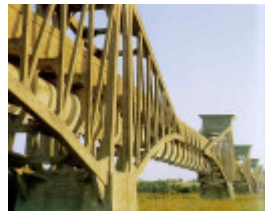
barwon river ovoid sewer aqueduct barwon river geelong site view publication
