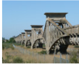
OVOID SEWER AQUEDUCT OVER BARWON RIVER SOHE 2008
