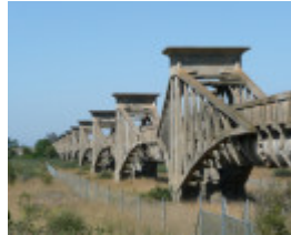
OVOID SEWER AQUEDUCT OVER BARWON RIVER SOHE 2008
