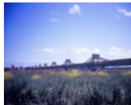
h00895 ovoid sewer aqueduct over barwon river south barwon geelong distant view she project 2004
