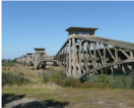
OVOID SEWER AQUEDUCT OVER BARWON RIVER SOHE 2008
