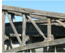
OVOID SEWER AQUEDUCT OVER BARWON RIVER SOHE 2008
