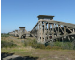
OVOID SEWER AQUEDUCT OVER BARWON RIVER SOHE 2008
