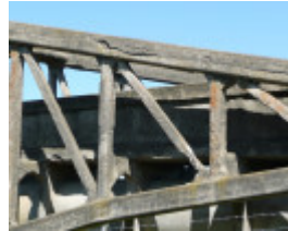
OVOID SEWER AQUEDUCT OVER BARWON RIVER SOHE 2008
