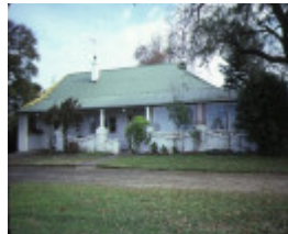
1 ellerslie pilmer street bacchus marsh front view homestead
