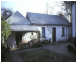
ellerslie pilmer street bacchus marsh front view cottage & coolroom
