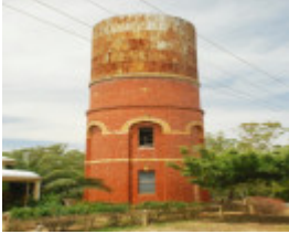
FORMER ELMORE WATER TOWER SOHE 2008
