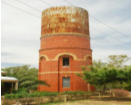
FORMER ELMORE WATER TOWER SOHE 2008
