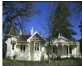
1 corio villa geelong front view
