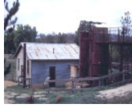
h01322 1 forest creek tourist gold mine castlemaine and chewton road castlemaine engine shed side elevation she project 2003
