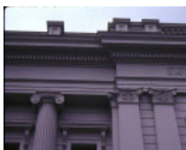
geelong town hall gheringhap street geelong column detail
