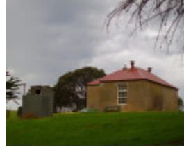
52774 School No 32 Lower Bridgewater 124
