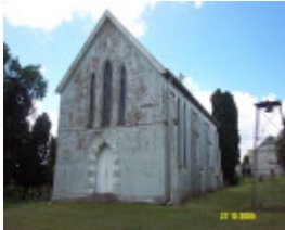
52940 St John s Anglican Digby 130
