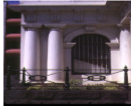
trustees chambers malop street geelong iron work
