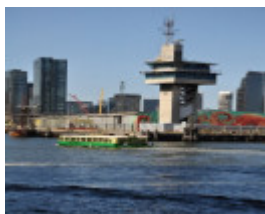
The Shipping Control Tower in 2024 prior to repair works
