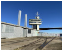
2025 Shipping Control Tower viewed from Victoria Dock - Photo - Heritage Victoria
