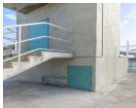
2025 Shipping Control Tower base - Photo - Development Victoria
