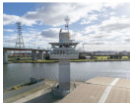
2025 Shipping Control Tower view from south Photo - Development Victoria
