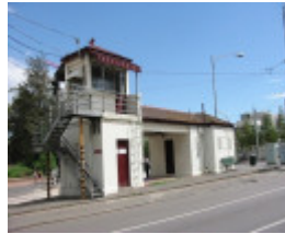
Swanston Street Tramway Signal Cabin February 2002
