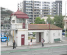
TRAMWAY SIGNAL CABIN, WAITING SHELTER AND CONVENIENCES SOHE 2008
