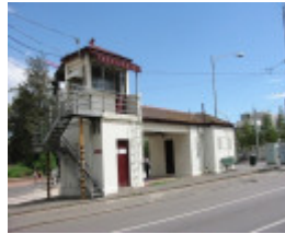
Swanston Street Tramway Signal Cabin February 2002
