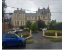
Maud Street Entrance
