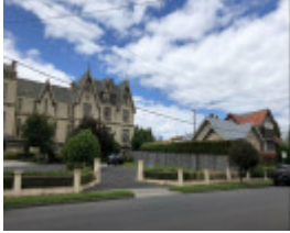
Maud Street elevation with bungalow at right
