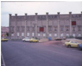
dennys lascelles wool stores geelong front view bow truss building demolished 1990
