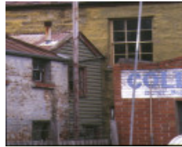
leyton & rochford moorabool street geelong rear buildings
