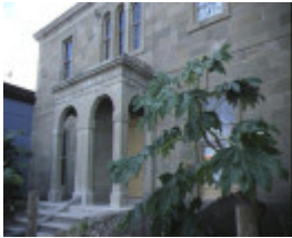
leyton & rochford moorabool street geelong entrance view
