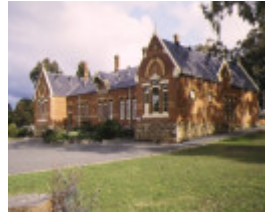
1 primary school number 1254 south west corner of high street maldon front view
