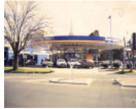
1 beaurepaire motor garage hargraves street bendigo front view
