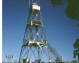
1 mount tarrengower lookout tower mount tarrengower maldon front view feb1997
