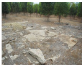
DEEP LEADS ELECTRIC COMMISSION POWER HOUSE SOHE 2008
