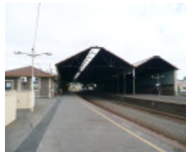
GEELONG RAILWAY STATION SOHE 2008
