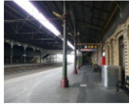
GEELONG RAILWAY STATION SOHE 2008
