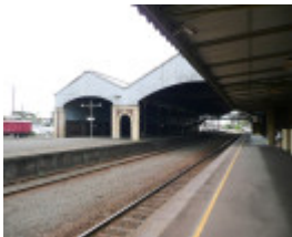
GEELONG RAILWAY STATION SOHE 2008
