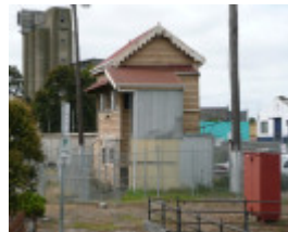
GEELONG RAILWAY STATION SOHE 2008
