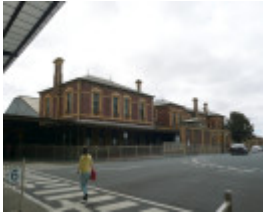
GEELONG RAILWAY STATION SOHE 2008
