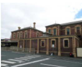
GEELONG RAILWAY STATION SOHE 2008
