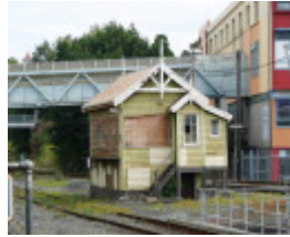
GEELONG RAILWAY STATION SOHE 2008
