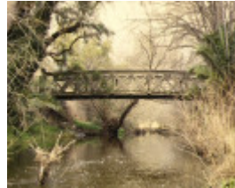
1 concrete truss footbridge over barkers creek castlemaine side view sep1997
