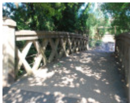
CONCRETE TRUSS FOOTBRIDGE SOHE 2008
