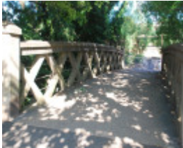
CONCRETE TRUSS FOOTBRIDGE SOHE 2008
