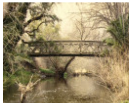
1 concrete truss footbridge over barkers creek castlemaine side view sep1997
