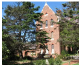
Wardell Building from nth west.jpg
