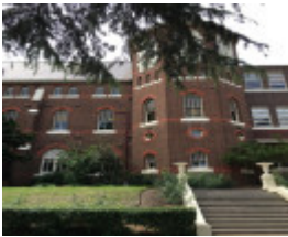
west side of Wardell Bldg.jpg
