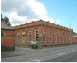
GAS REGULATING HOUSE SOHE 2008
