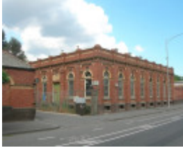
GAS REGULATING HOUSE SOHE 2008
