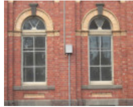
GAS REGULATING HOUSE SOHE 2008
