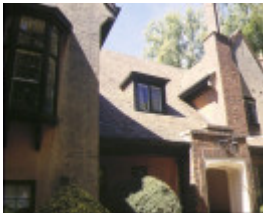
1 little milton albany road toorak front view feb1998
