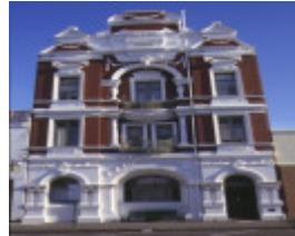
1 former royal hotel nelson place williamstown front view sep1998
