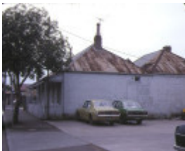
former harp inn packington street geelong west side view jul1984
