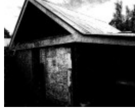
Detached store or early house from the south-east, showing shingle roof under added gabled roof
