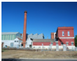
THOMPSONS KELLY & LEWIS ENGINEERING WORKS SOHE 2008
