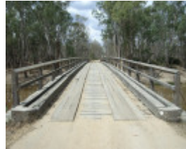
CONDIDORIOS BRIDGE SOHE 2008
