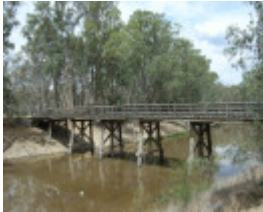
CONDIDORIOS BRIDGE SOHE 2008
