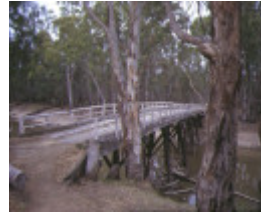
1 condidorios bridge koondrook
