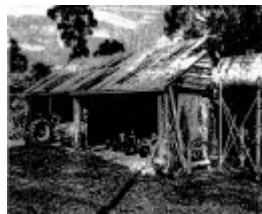
12.11 - Tregowan Cottage 08 - Shire of Whittlesea Heritage Study 1991
