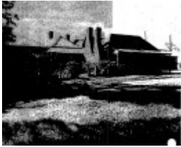
12.11 - Tregowan Cottage - Shire of Whittlesea Heritage Study 1991
