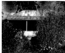
12.11 - Tregowan Cottage 05 - Shire of Whittlesea Heritage Study 1991
