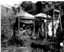
12.11 - Tregowan Cottage 06 - Shire of Whittlesea Heritage Study 1991
