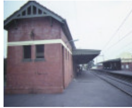
1 glenferrie railway station hawthorn station building jun1984
