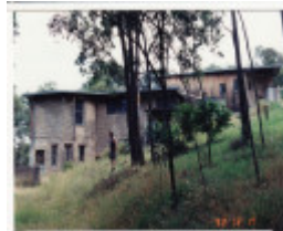
Frank Werther Residence off Barreenong Rd Colour 3 - Shire of Eltham Heritage Study 1992
