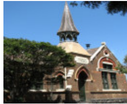
GLENFERRIE PRIMARY SCHOOL (PRIMARY SCHOOL NO.1508) SOHE 2008
