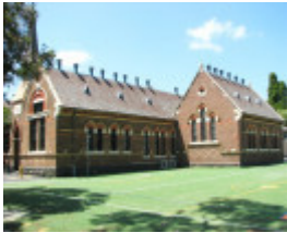
GLENFERRIE PRIMARY SCHOOL (PRIMARY SCHOOL NO.1508) SOHE 2008
