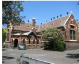
GLENFERRIE PRIMARY SCHOOL (PRIMARY SCHOOL NO.1508) SOHE 2008
