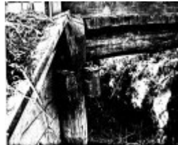
33 - Timber Trestle Road Bridge over Arthurs Creek_03 - Shire of Eltham Heritage Study 1992
