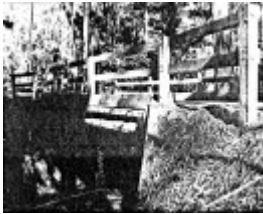
33 - Timber Trestle Road Bridge over Arthurs Creek - Shire of Eltham Heritage Study 1992
