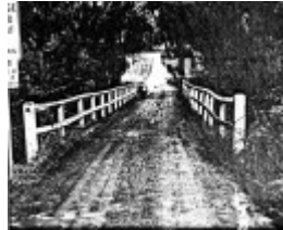
34 - Timber Trestle Road Bridge Chapel Lane - Shire of Eltham Heritage Study 1992
