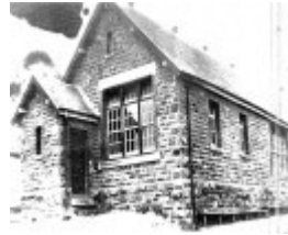
50 - Eltham Primary School Dalton St - Early 20th century photograph taken after the installation of larger windows, a process undertaken at many Victorian State Schools at that time. Note the smaller windows, which are presumably original (ELHPC No.642)
