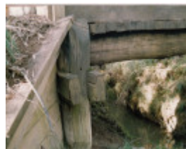
Timber Trestle Bridge Arthurs Creek Eagles Nest Rd Colour 5 - Shire of Eltham Heritage Study 1992
