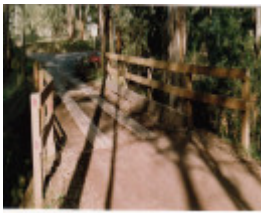
Timber Trestle Bridge Arthurs Creek Eagles Nest Rd Colour 4 - Shire of Eltham Heritage Study 1992
