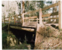
Timber Trestle Bridge Arthurs Creek Eagles Nest Rd Colour 3 - Shire of Eltham Heritage Study 1992
