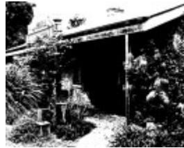
62 - Former Wellers Pub at Pitman Cnr Kangaroo Ground_02 - Shire of Eltham Heritage Study 1992
