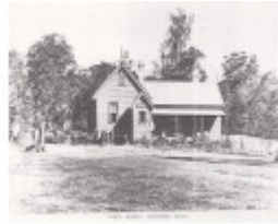
Kangaroo Primary State School Elth Yarr Glen Rd Black & White 2 - Shire of Eltham Heritage Study 1992
