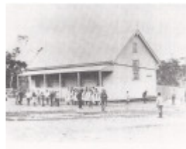
Kangaroo Primary State School Elth Yarr Glen Rd Black & White 3 - Shire of Eltham Heritage Study 1992
