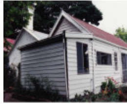
Garden Hill Shearing Shed Elth Yarra Glen Rd Colour 11 - Shire of Eltham Heritage Study 1992
