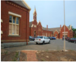
PRIMARY SCHOOL NO. 1566 SOHE 2008
