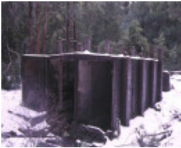
1 spring creek mill & kilns mt samaria seasoning kilns
