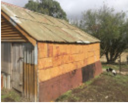
2017, shed, kerosene can cladding.jpg
